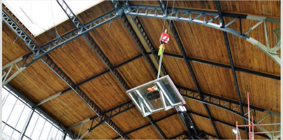
Colt Firelight ventilator being installed into the roof of Gare Maritime Railway Station.
