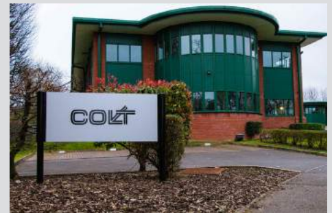
New Colt House in Petersfield, UK.
