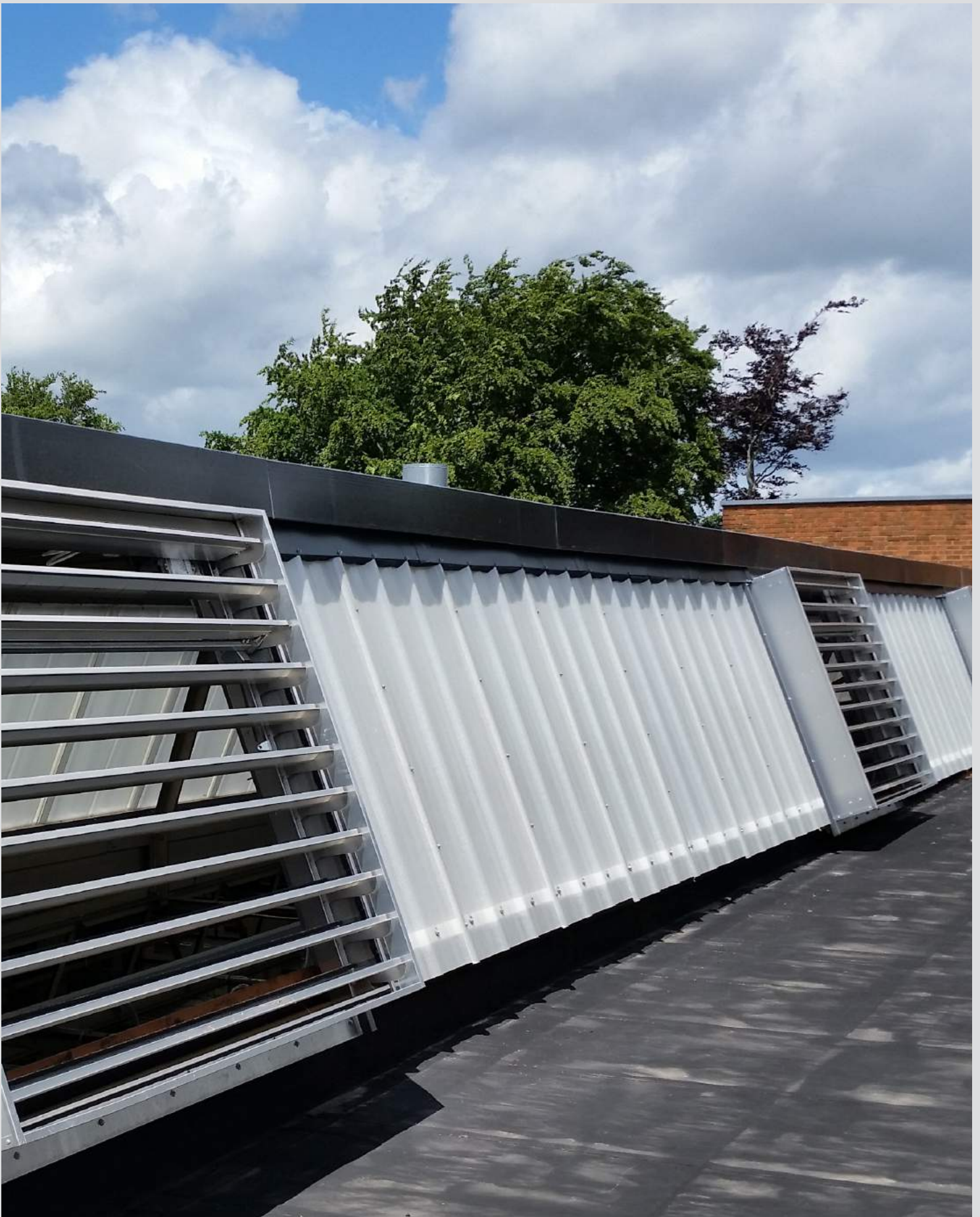
72 Seefire ventilators installed for natural ventilation and extraction of hot air to prevent overheating issues at Carlisle Fluid Technologies in Bournemouth, UK. This was to replace the original ventilation system, also provided by Colt, over 40 years ago.
